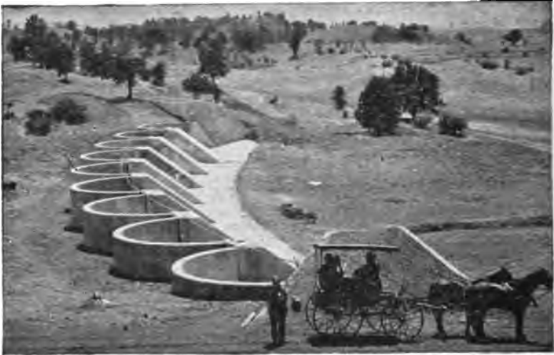
FIG. 242.—East Park Reservoir Spillway, Orland Project.
